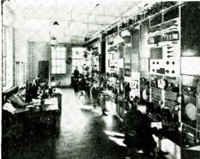
General Control Room, N. Y., supervises the nets. (Bell Tel. Co.)
